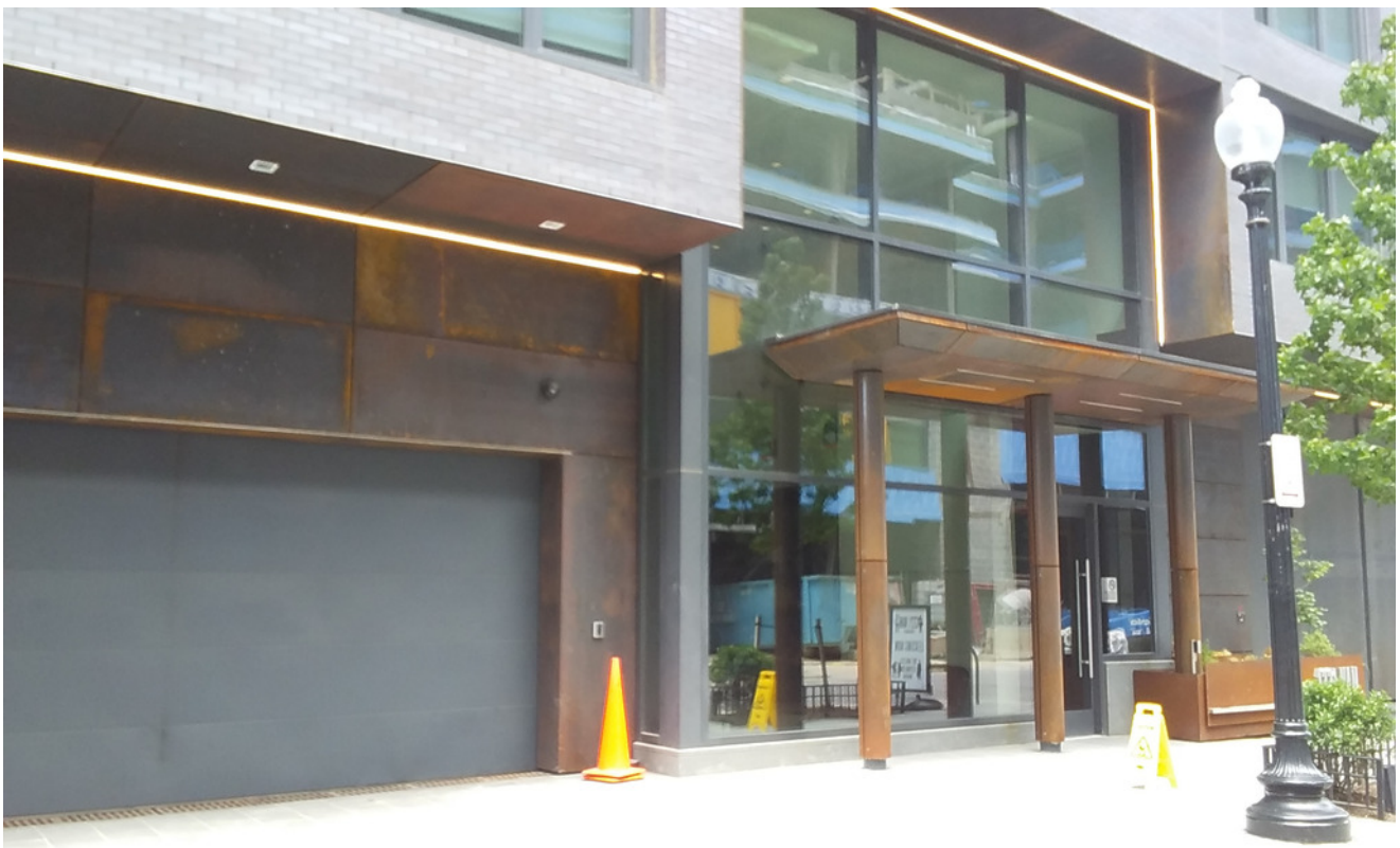
The protective patina of the Corten plate gives the building a weathered look. Material was even custom fit to shape the canopy and support poles of the entrance to the building. (photo: TSI Corporations)
